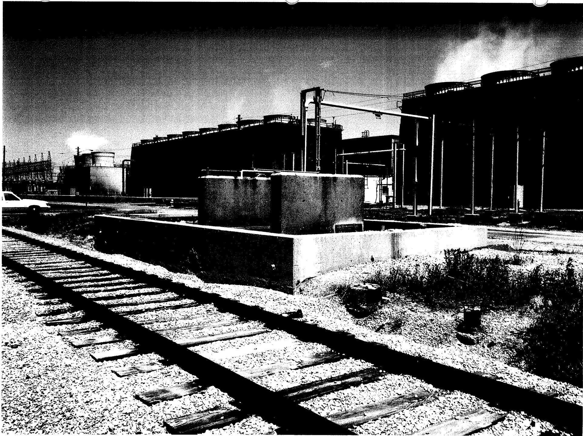
77. C-634-B H2S04 Storage Tank Figure EI.4. Photograph of SWMU 77
