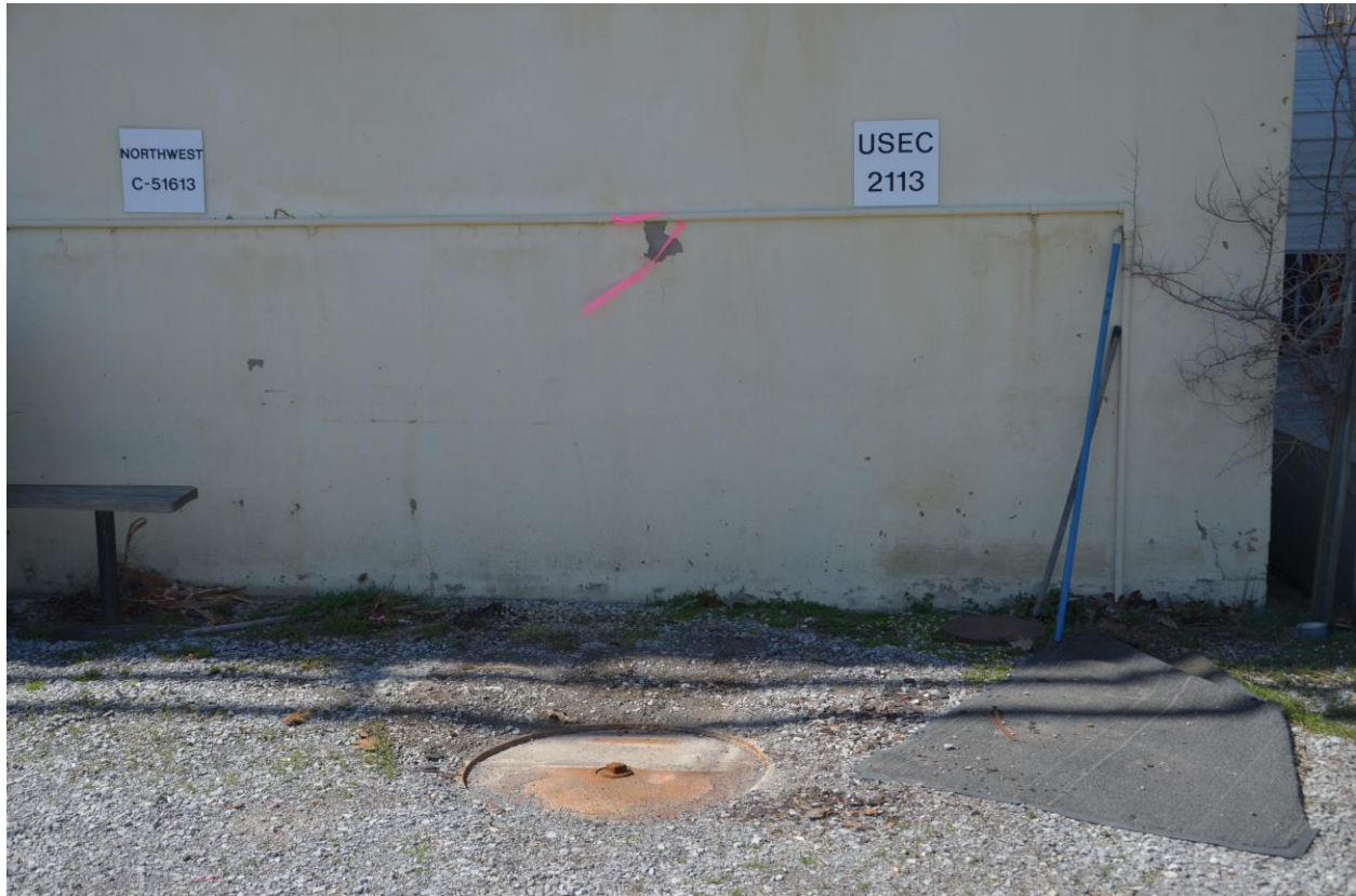
Figure 1.1. SWMU 27, C-722 Acid Neutralization Tank, Northeast Corner of C-720
