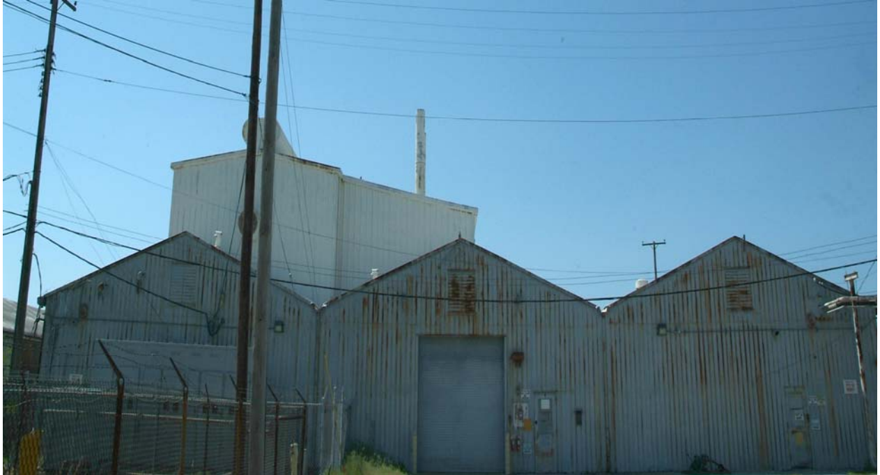
Figure 2. Exterior of the C-746-A East End Smelter
