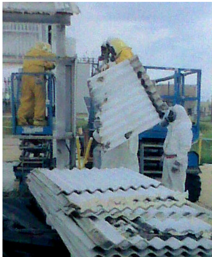
Figure A.5. Transite Siding Removal and Packaging
