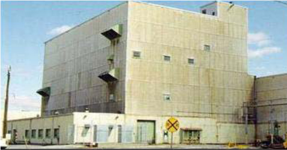
Figure 2. Exterior of the C-410 Complex
