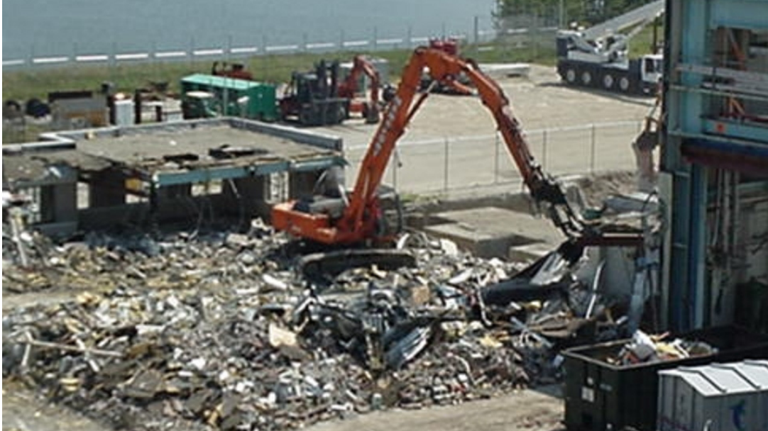
Figure A.6. Building Demolition Using “Long Reach” Excavator with Shear Attachment
