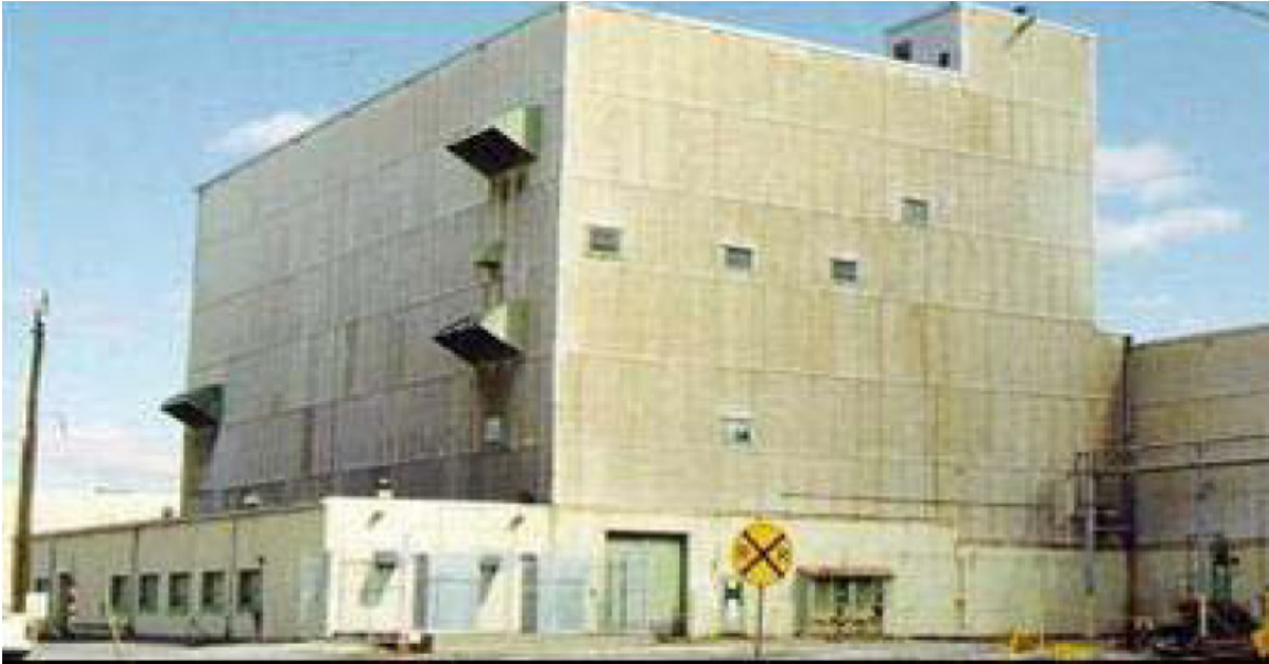
Figure A.2. Exterior of the C-410 Complex
