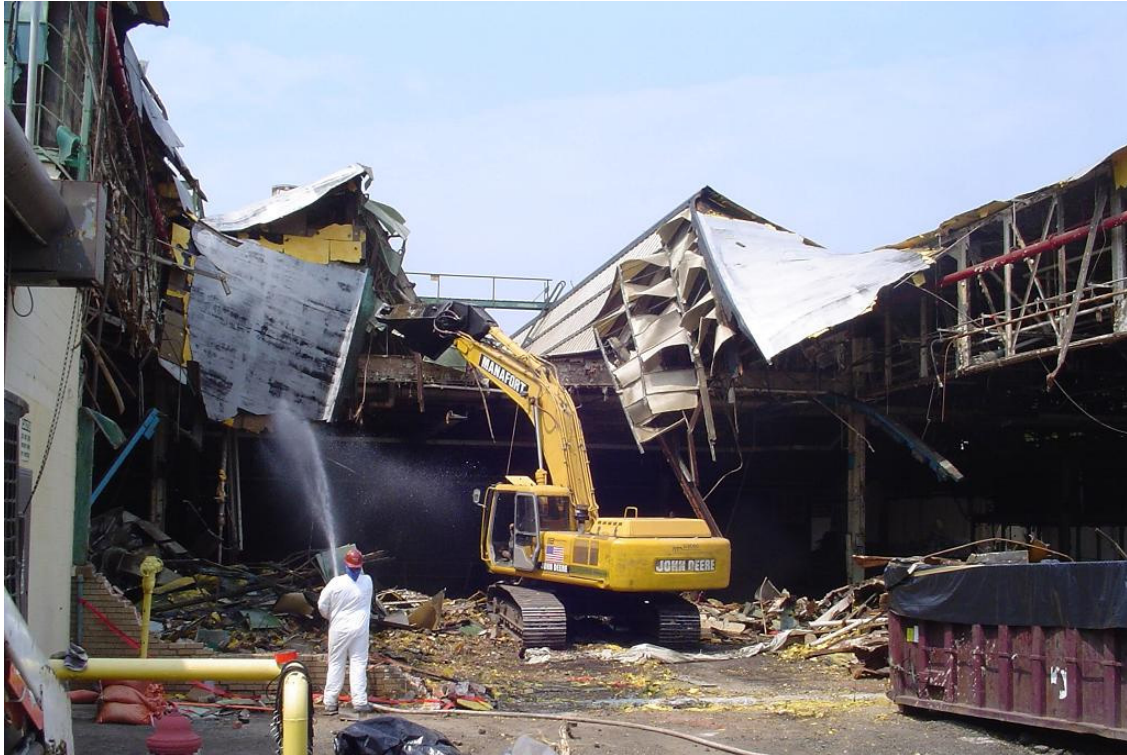
Figure A.3. Building Structure and Roof Demolition (Shear and Fugitive Dust Control)
