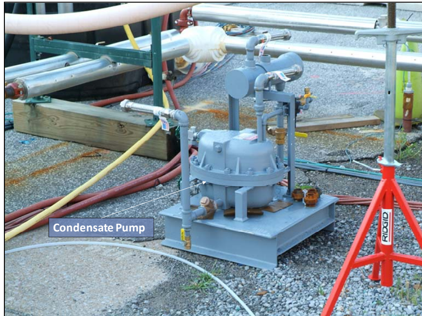
Figure 29. Condensate Pump
