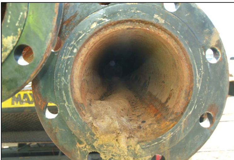
Figure 25. Sediment in the Vapor Extraction Header
