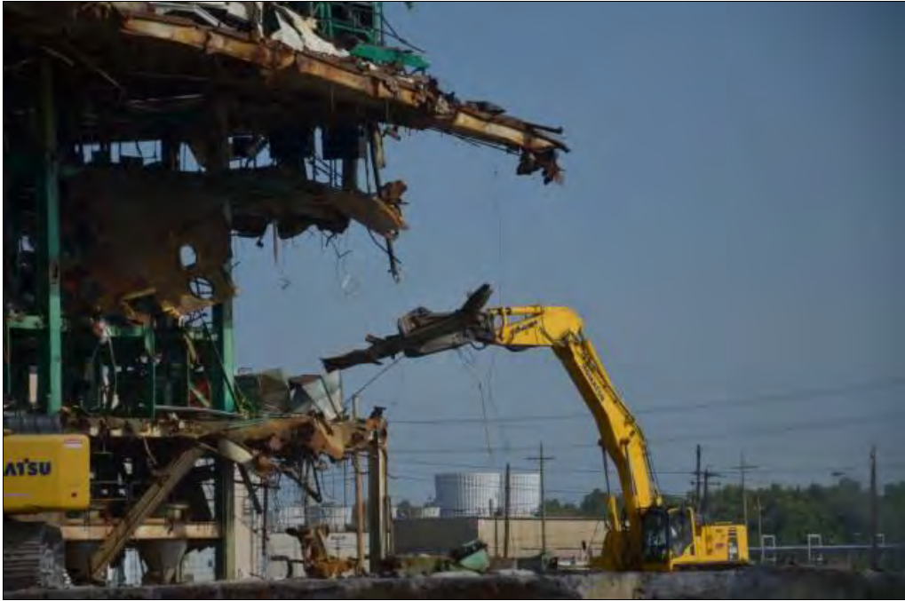
Figure A.5. Hydraulic Shears Mounted on an Excavator for Demolition Activities
