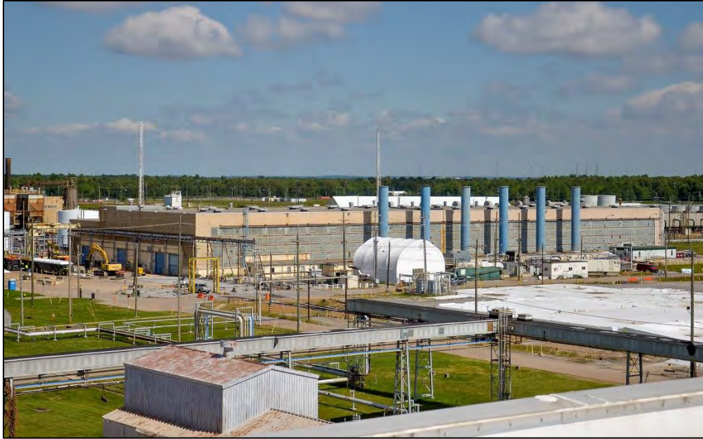
Figure A.2. Exterior of the C-400 Cleaning Building Looking to the Northwest
