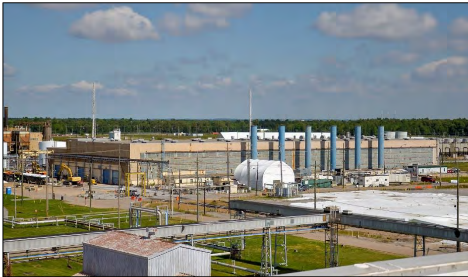
Figure 2. Exterior of the C-400 Cleaning Building Looking to the Northwest
