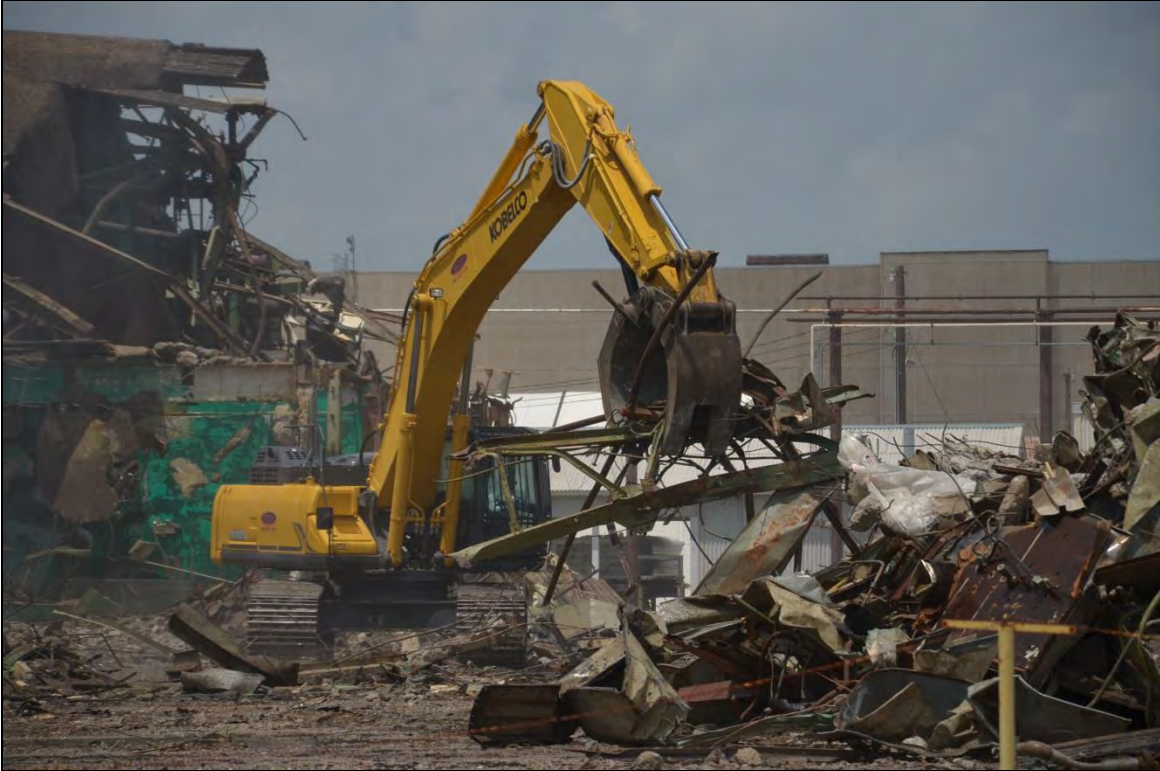
Figure A.8. Hydraulic Grapple Mounted on an Excavator for Loading Demolition Debris on to Conveyance
