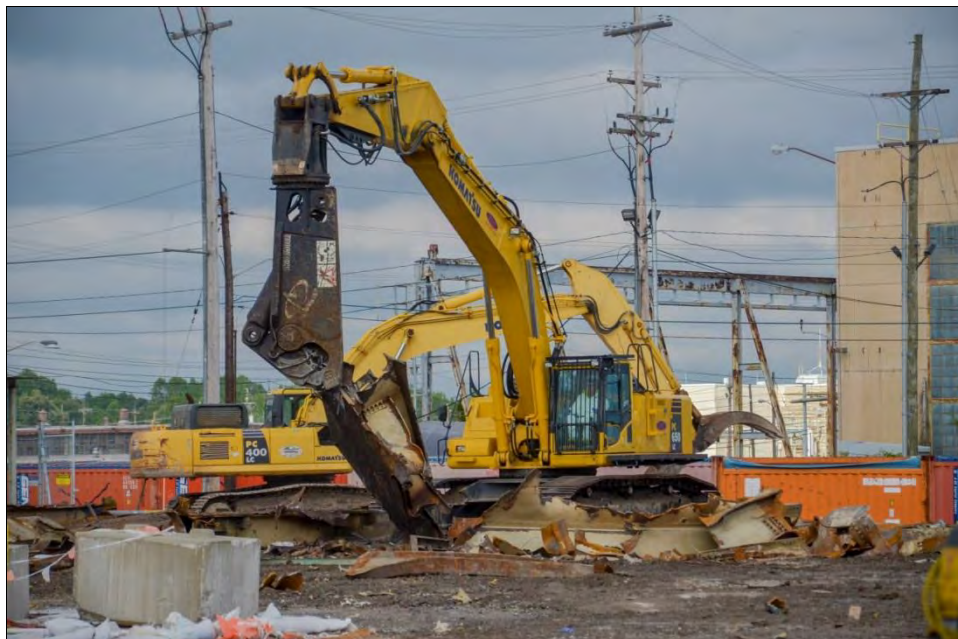
Figure A.7. Hydraulic Shears Mounted on an Excavator for Size-reducing Demolition Debris
