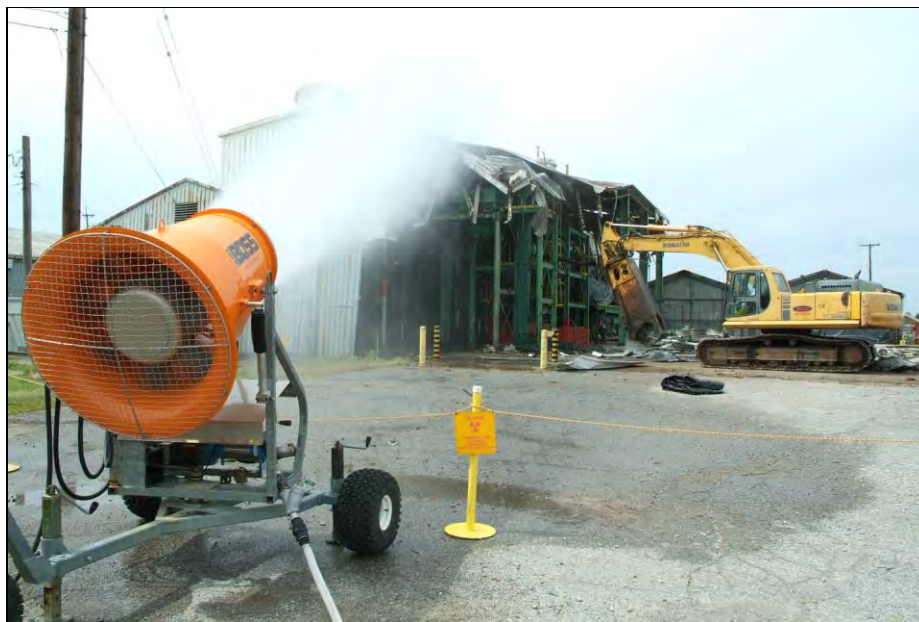
Figure A.4. Misting Unit Used for Dust Suppression during Demolition
