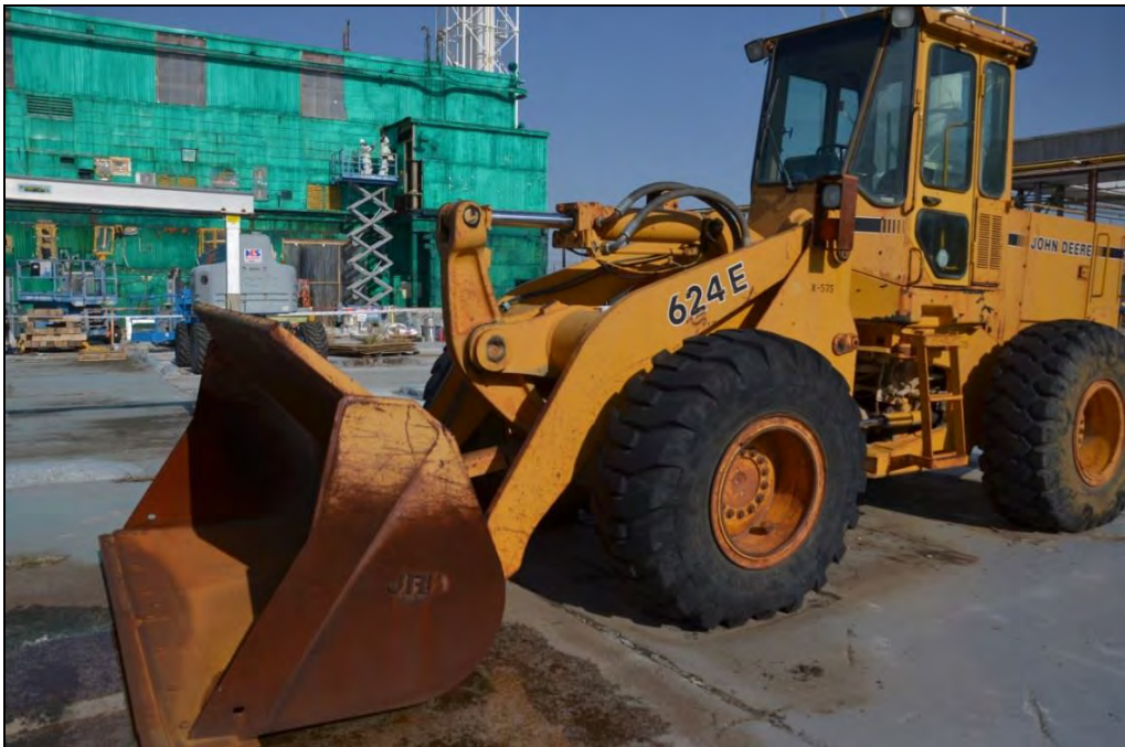
Figure A.6 Front End Loader Used to Move Debris within the Demolition Site
