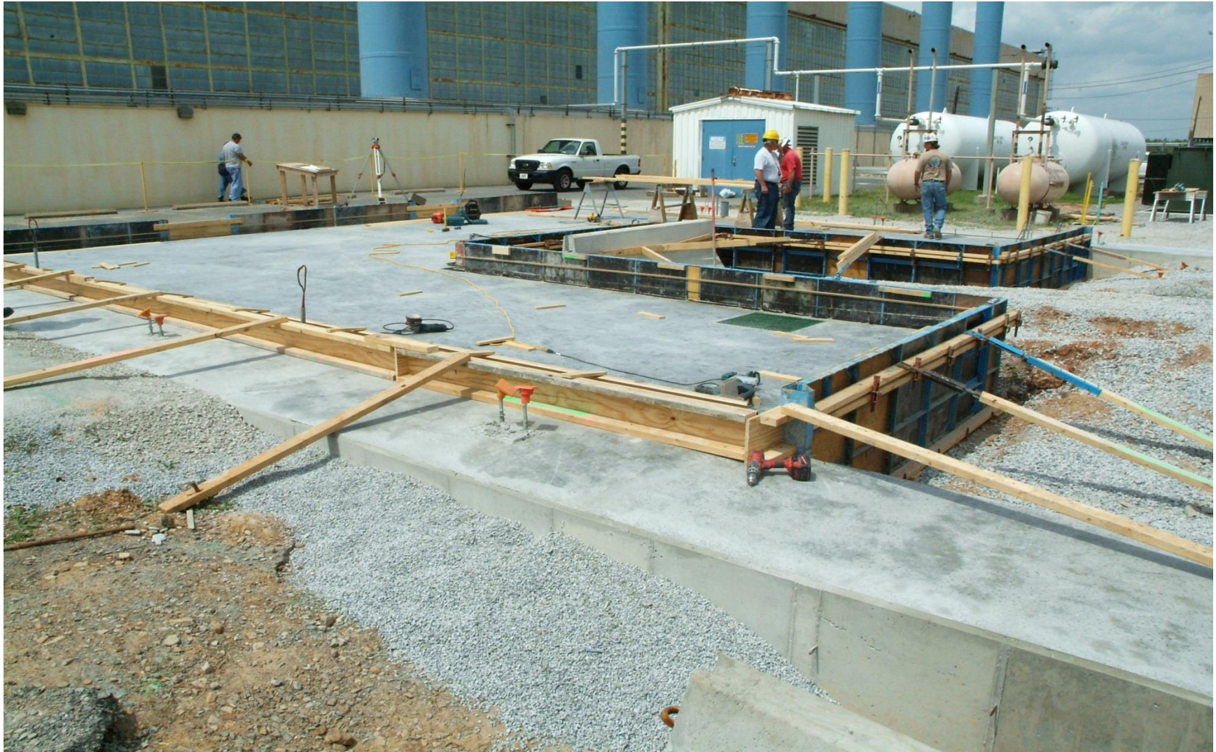
Figure 4.2. Foundation Construction for Treatment Equipment
