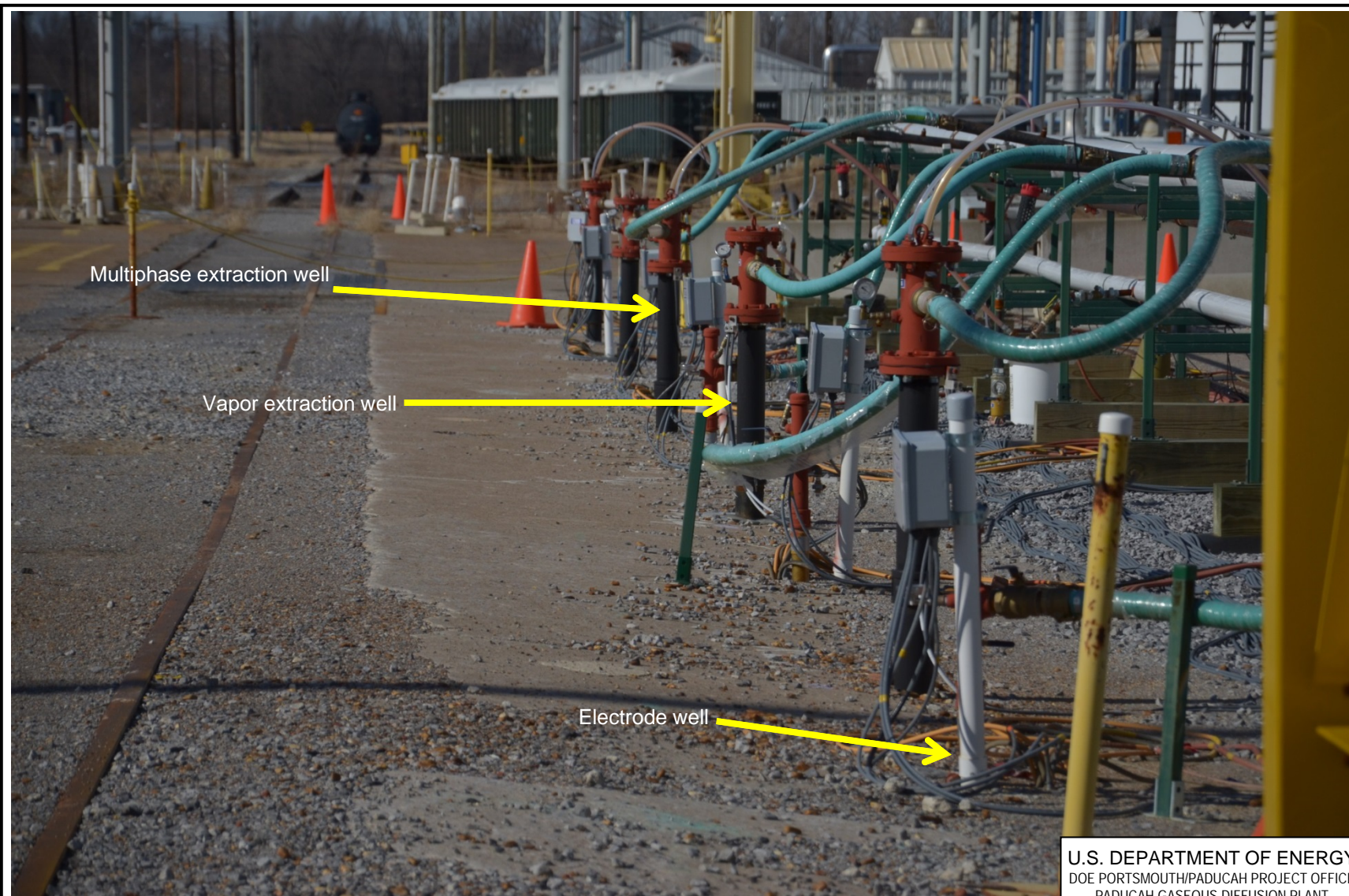
Figure 5.11. C-400 Phase IIa ERH Wellfield
