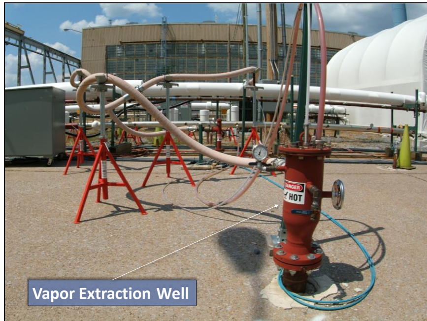
Figure 4.16. Vapor Extraction Well
