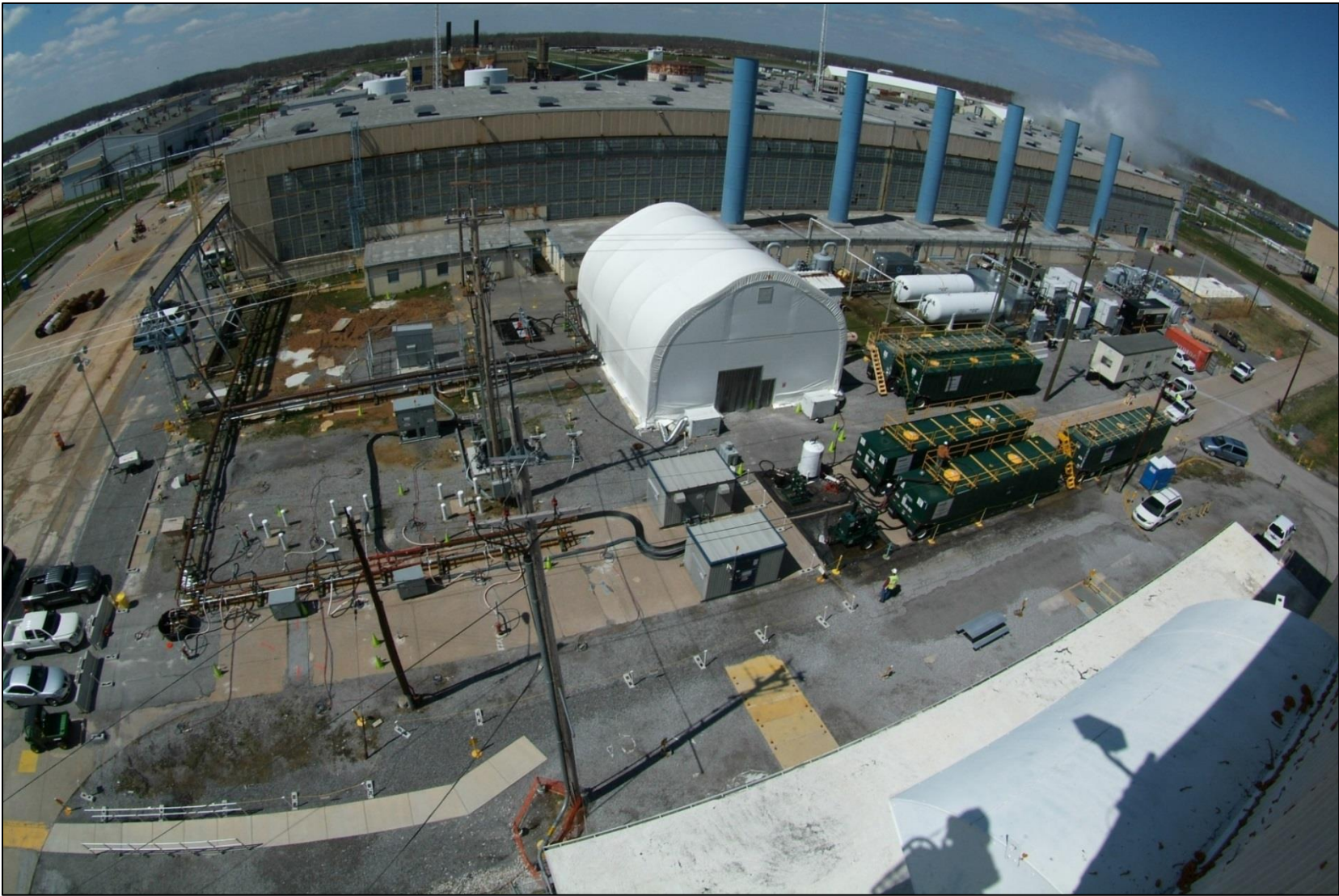
Figure 4.7. Picture of Groundwater/Vapor Treatment System Area
