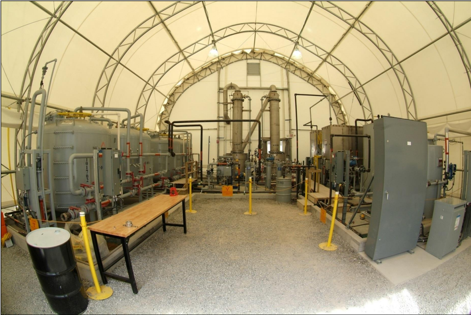
Figure 4.8. Treatment Equipment (Tent Area)
