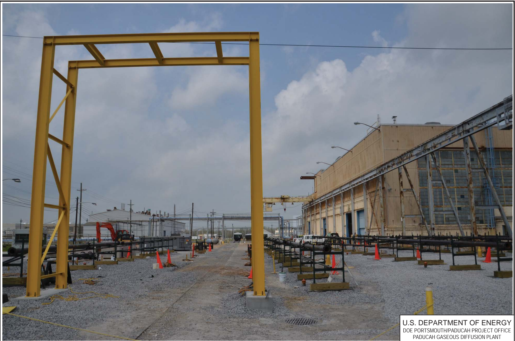
Figure 5.15. C-400 Phase IIa Construction of ERH Laterals
