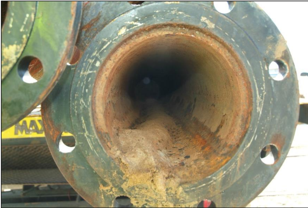
Figure 4.23. Sediment in the Vapor Extraction Header
