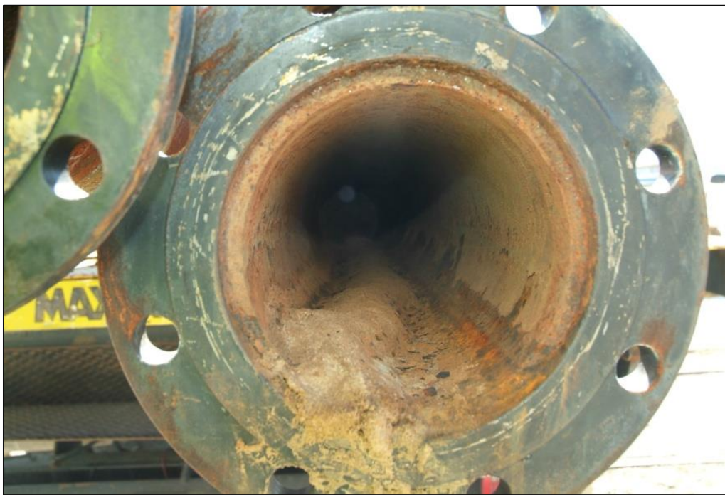
Figure 4.22. Sediment in the Vapor Extraction Header
