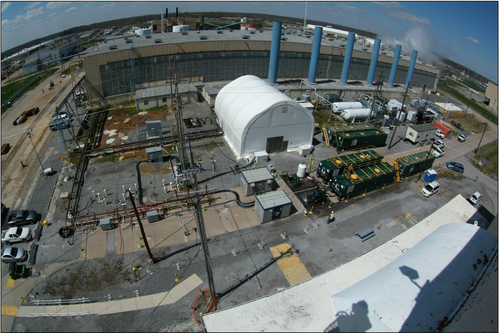
Figure 4.6. Picture of Groundwater/Vapor Treatment System Area
