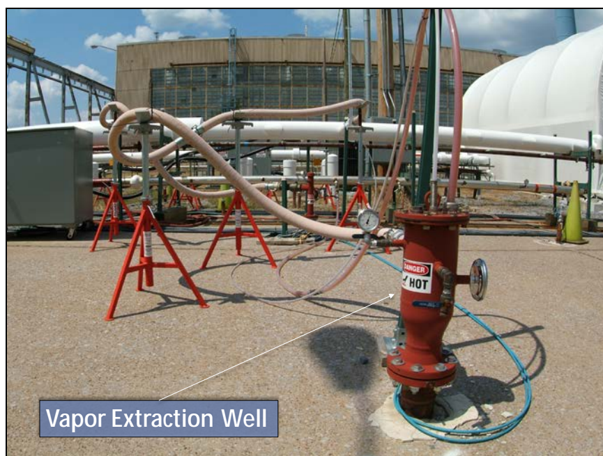
Figure 4.15. Vapor Extraction Well
