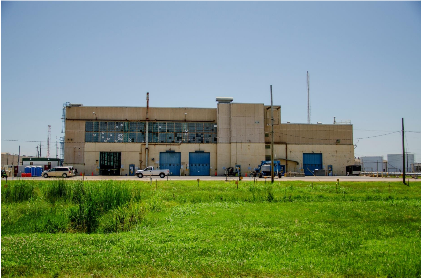
Figure 8. North Facade of the C-400 Cleaning Building Facing South (2018)
