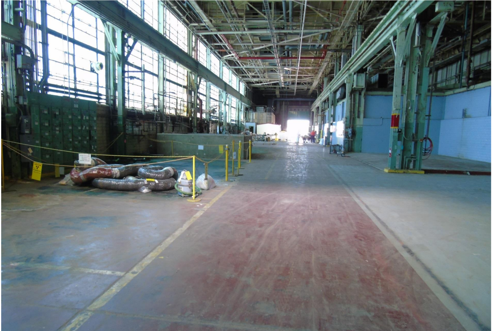
Figure 11. West Side Interior of the C-400 Cleaning Building Facing North (2017)
