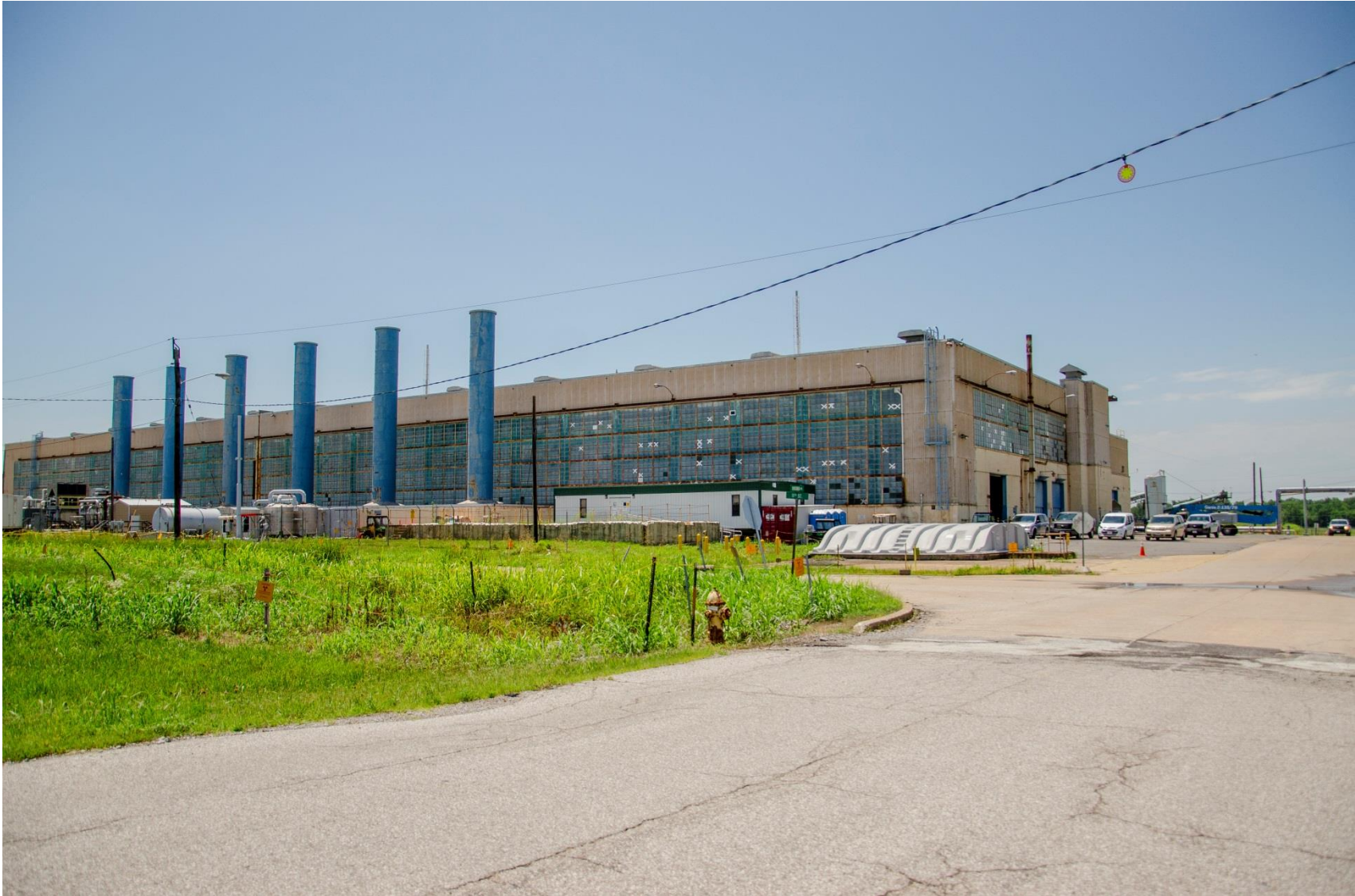
Figure 3. Northeast Corner of the C-400 Cleaning Building Facing Southwest (2018)
