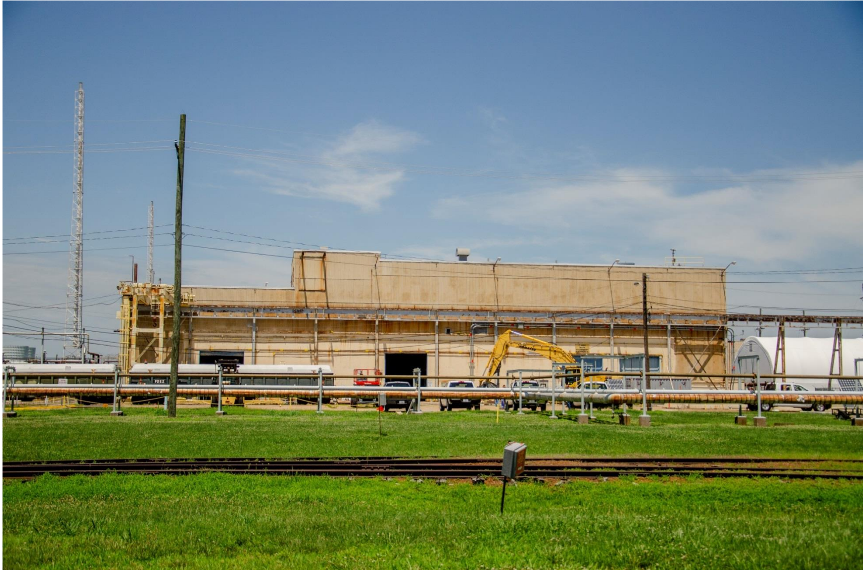
Figure 5. South Facade of the C-400 Cleaning Building Facing North (2018)
