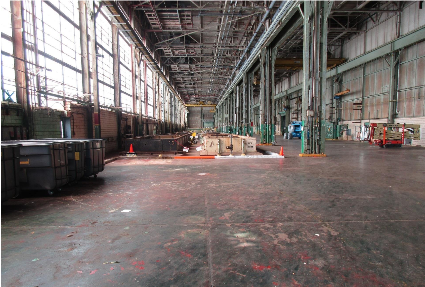
Figure 10. East Side Interior of the C-400 Cleaning Building Facing South (2017)
