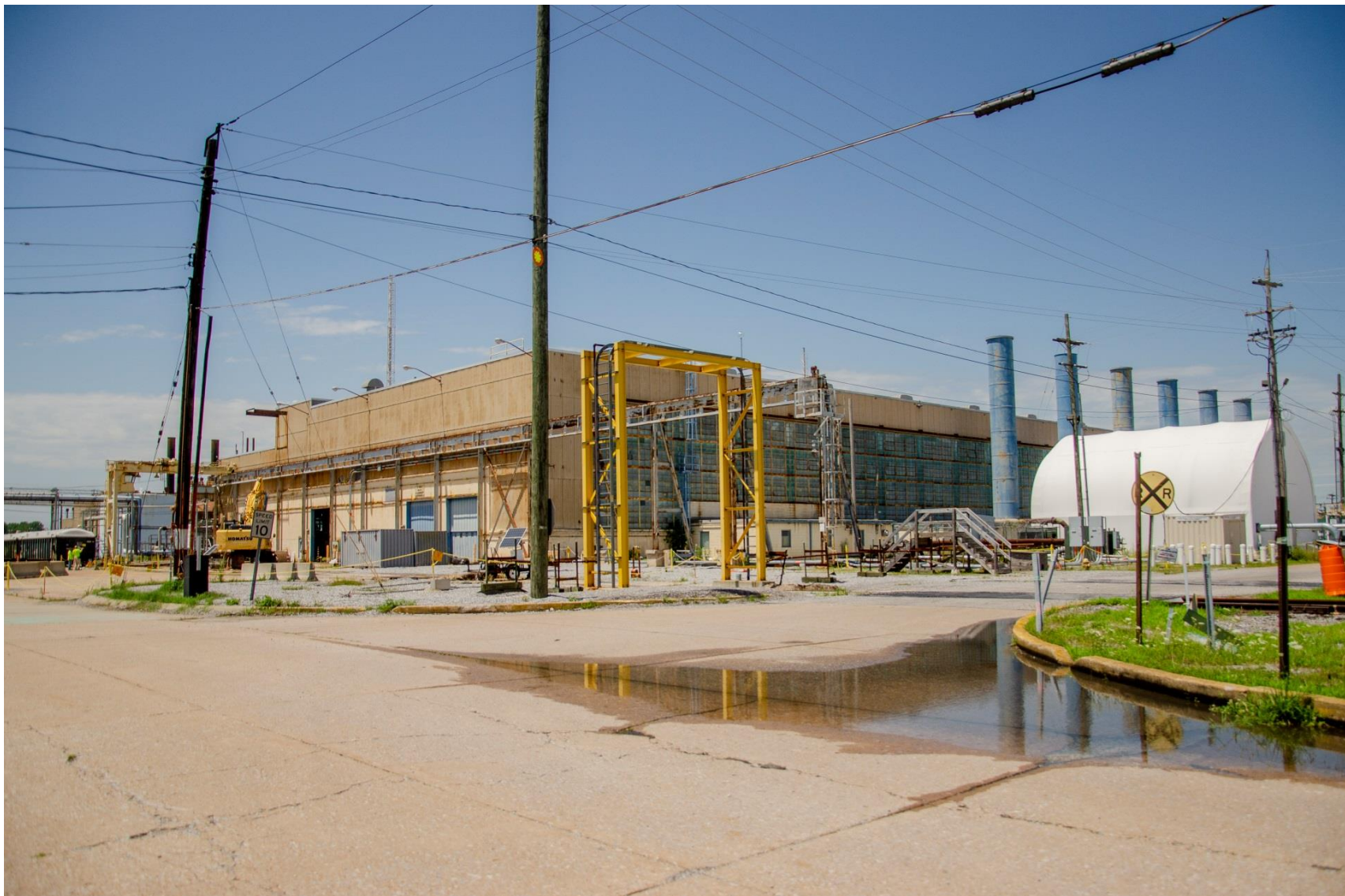
Figure 4. Southeast Corner of the C-400 Cleaning Building Facing Northwest (2018)
