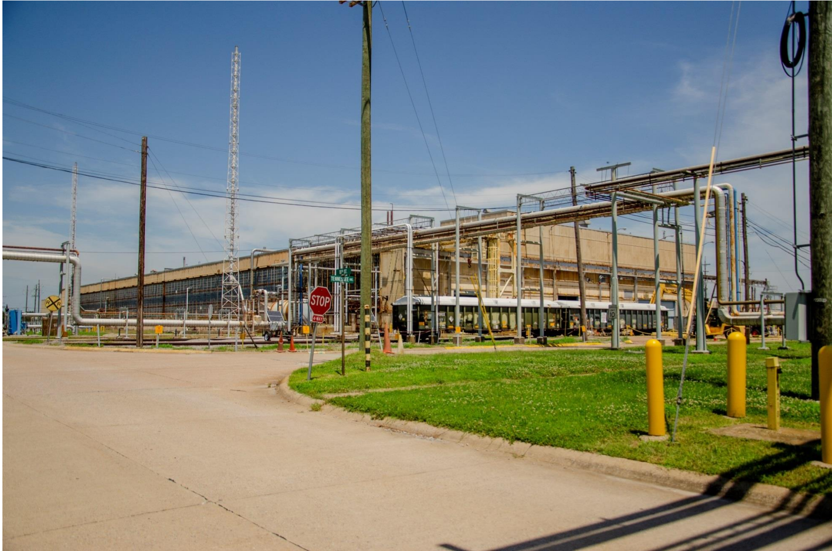
Figure 6. Southwest Corner of the C-400 Cleaning Building Facing Northeast (2018)
