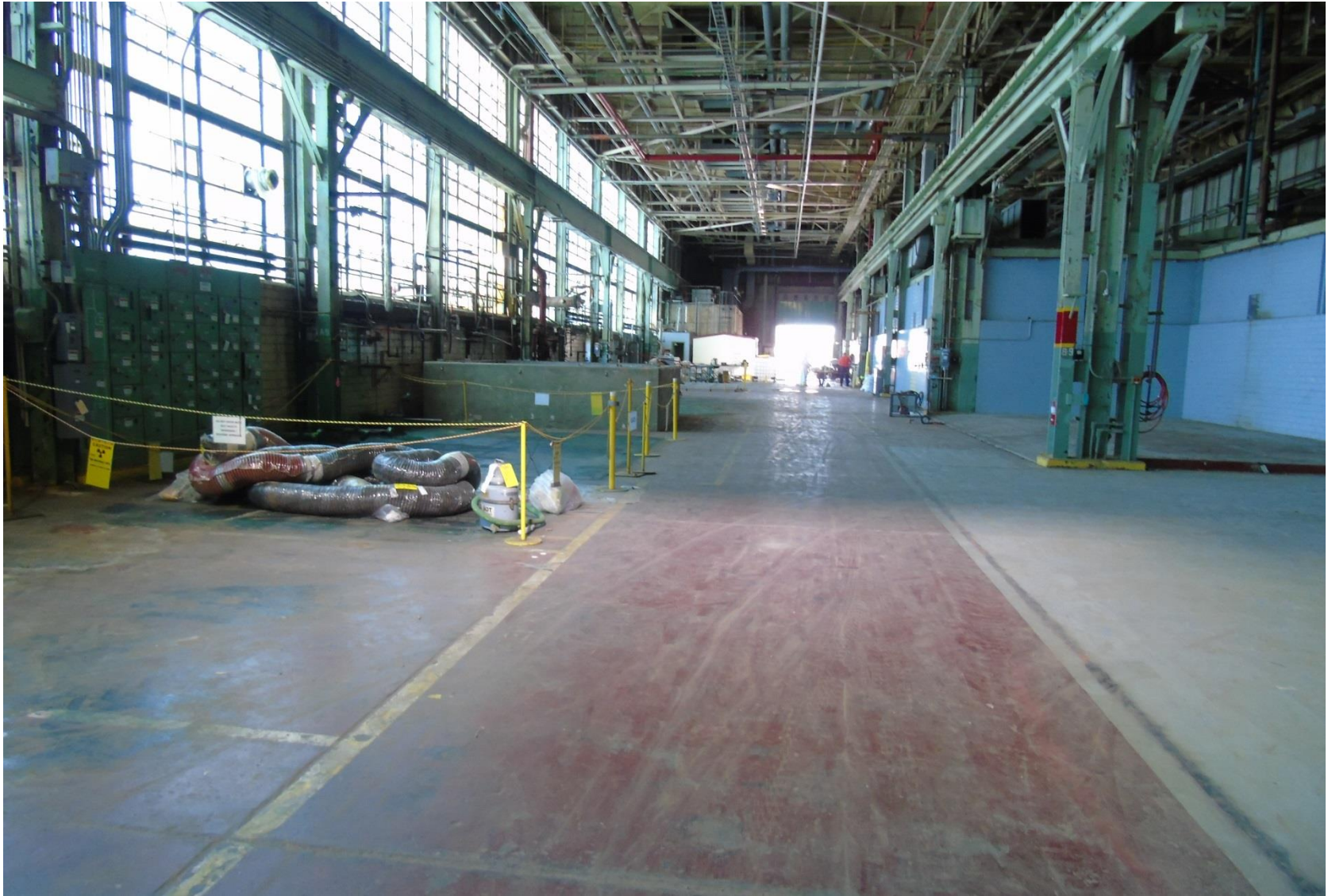
Figure 8. West Side Interior of the C-400 Cleaning Building Facing North (2017)
