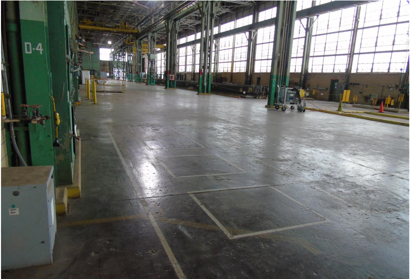
Figure 6. East Side Interior of the C-400 Cleaning Building Facing North (2017)
