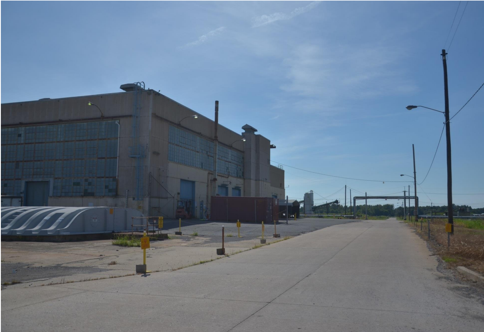
Figure 3. Northeast Corner of the C-400 Cleaning Building Facing West (2016)
