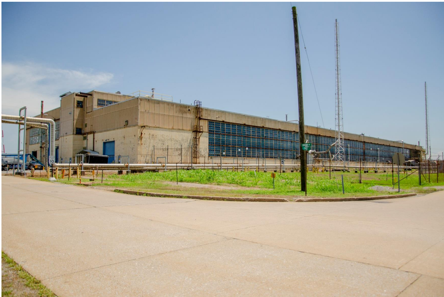
Figure 7. Northwest Corner of the C-400 Cleaning Building Facing Southeast (2018)
