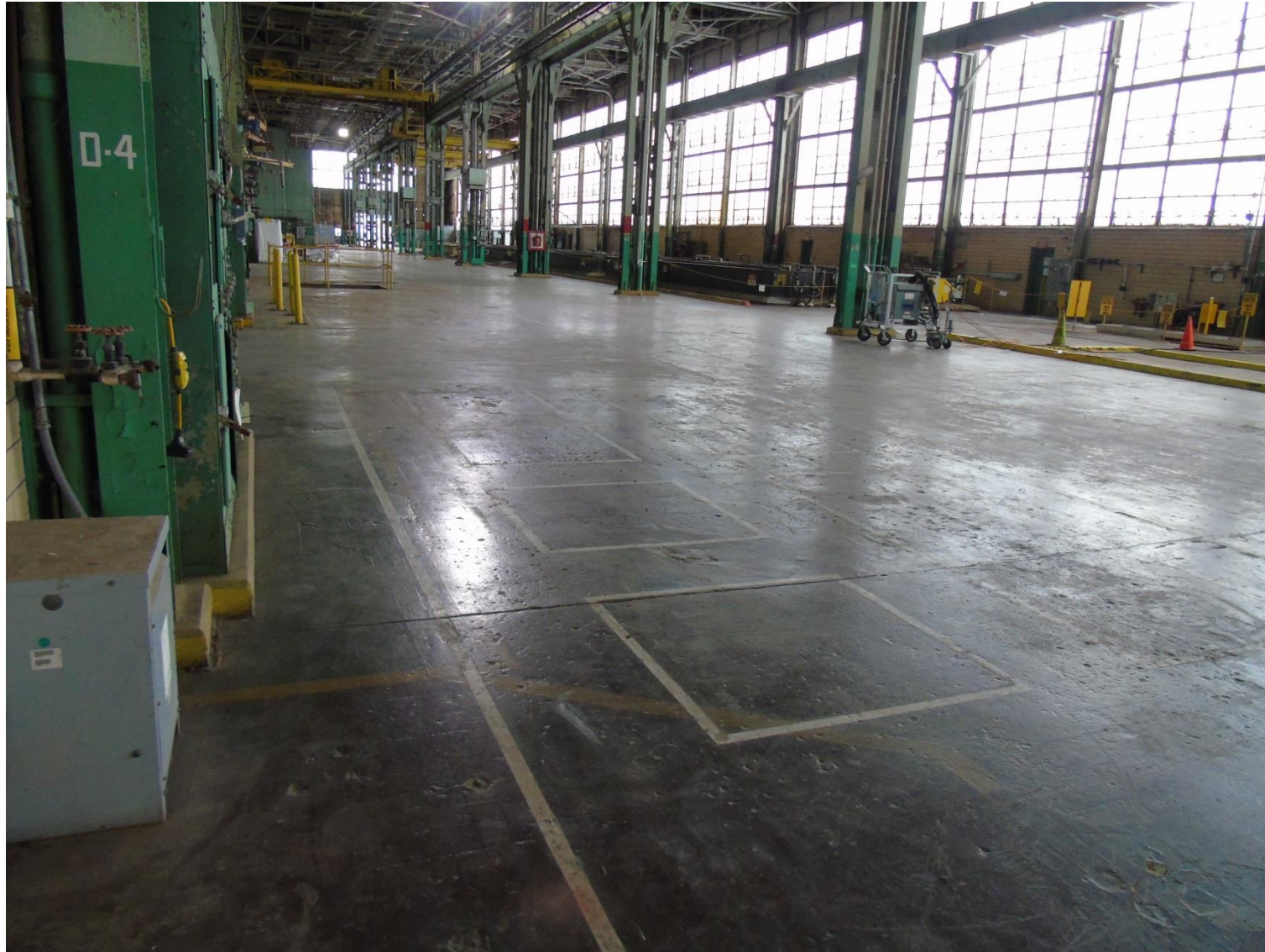
Figure 9. East Side Interior of the C-400 Cleaning Building Facing North (2017)
