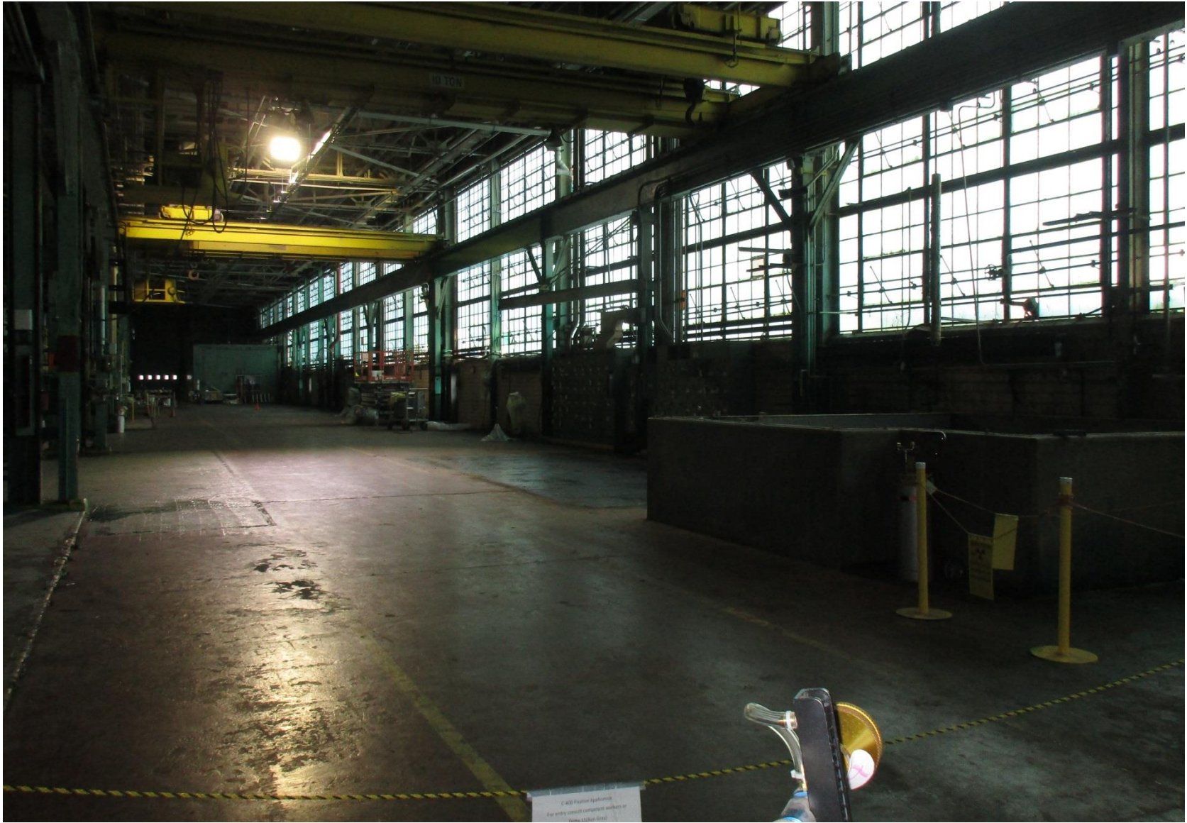
Figure 12. West Side Interior of the C-400 Cleaning Building Facing South (2017)
