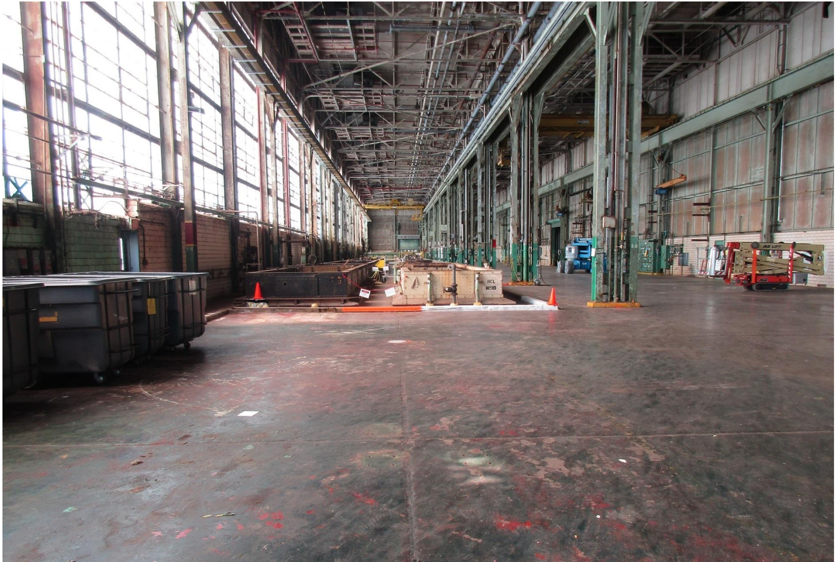
Figure 7. East Side Interior of the C-400 Cleaning Building Facing South (2017)
