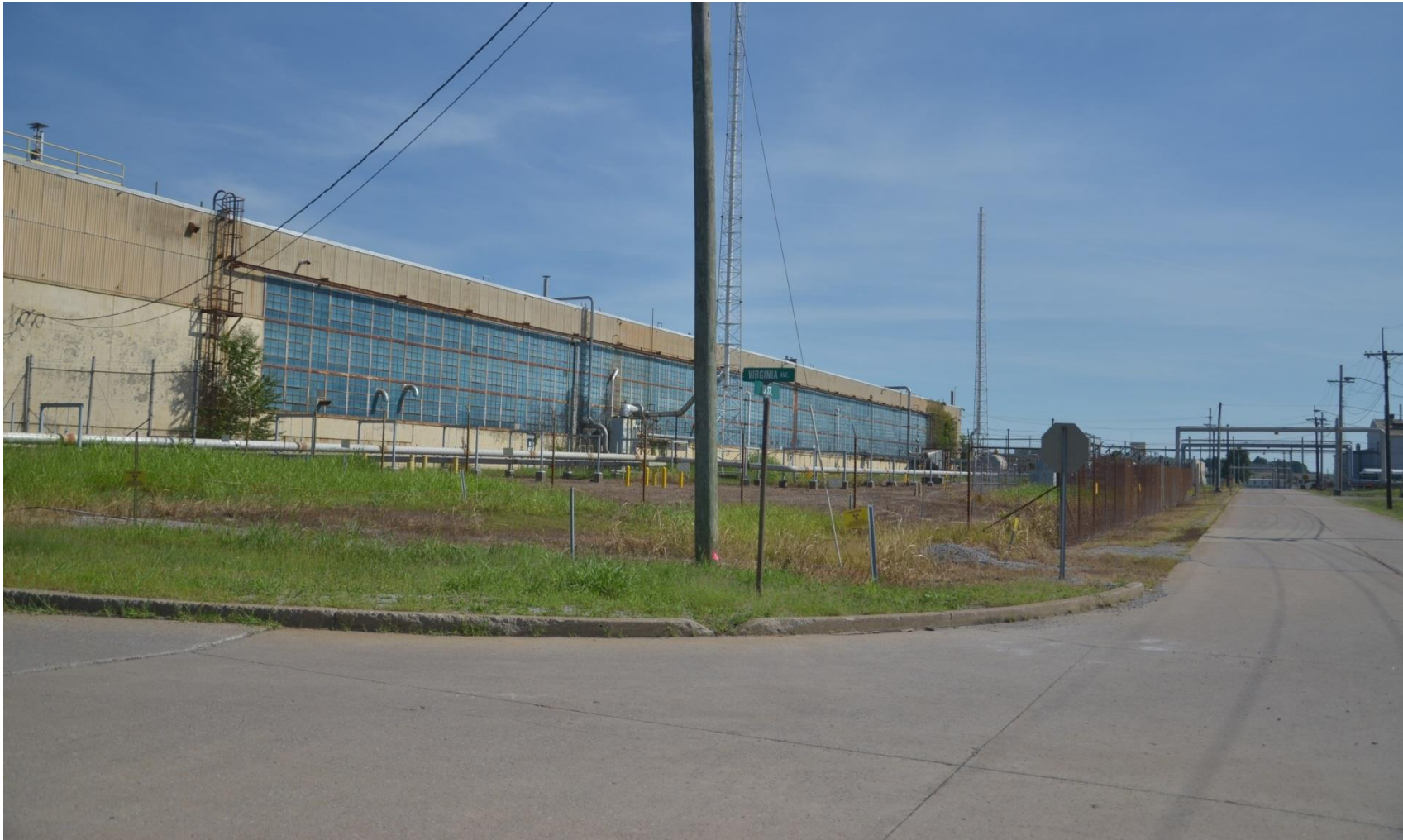
Figure 5. West Side of the C-400 Cleaning Building Facing Southeast (2017)
