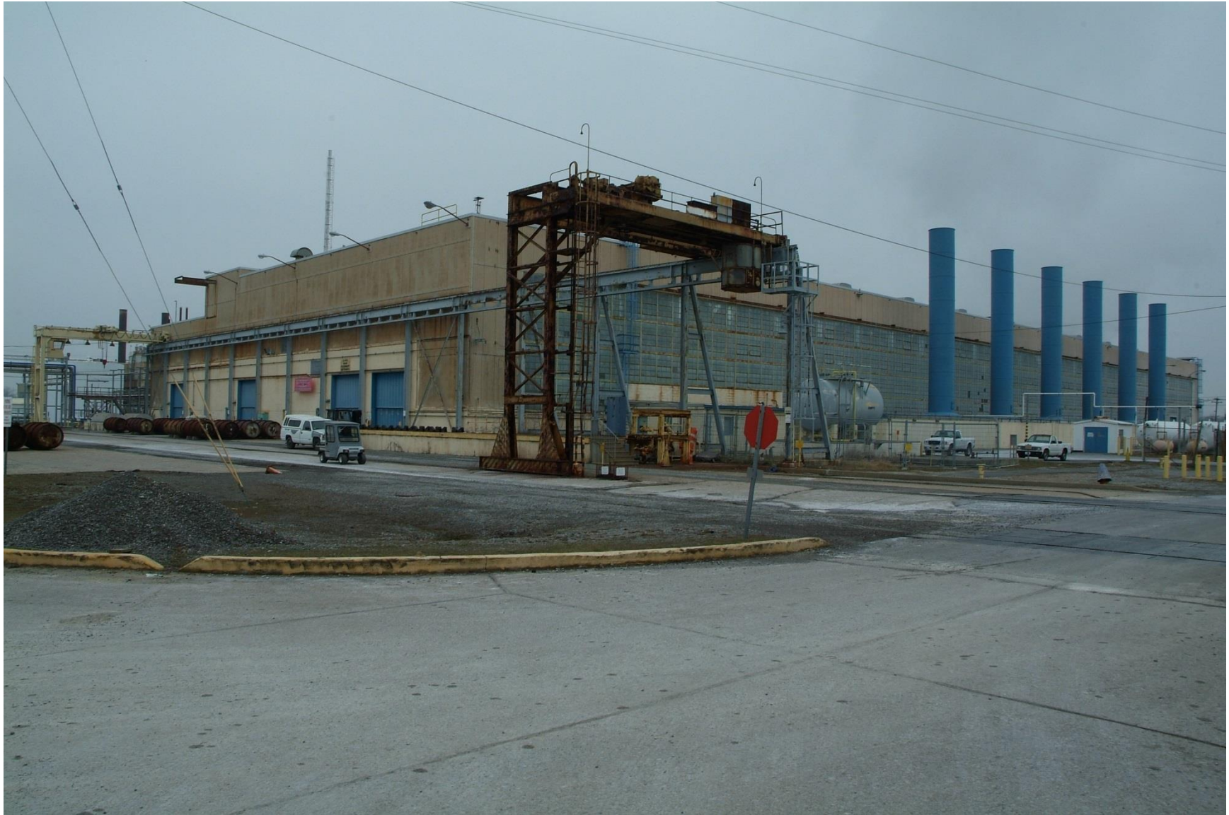
Figure 4. Southeast Corner of the C-400 Cleaning Building Facing Northwest (2008)
