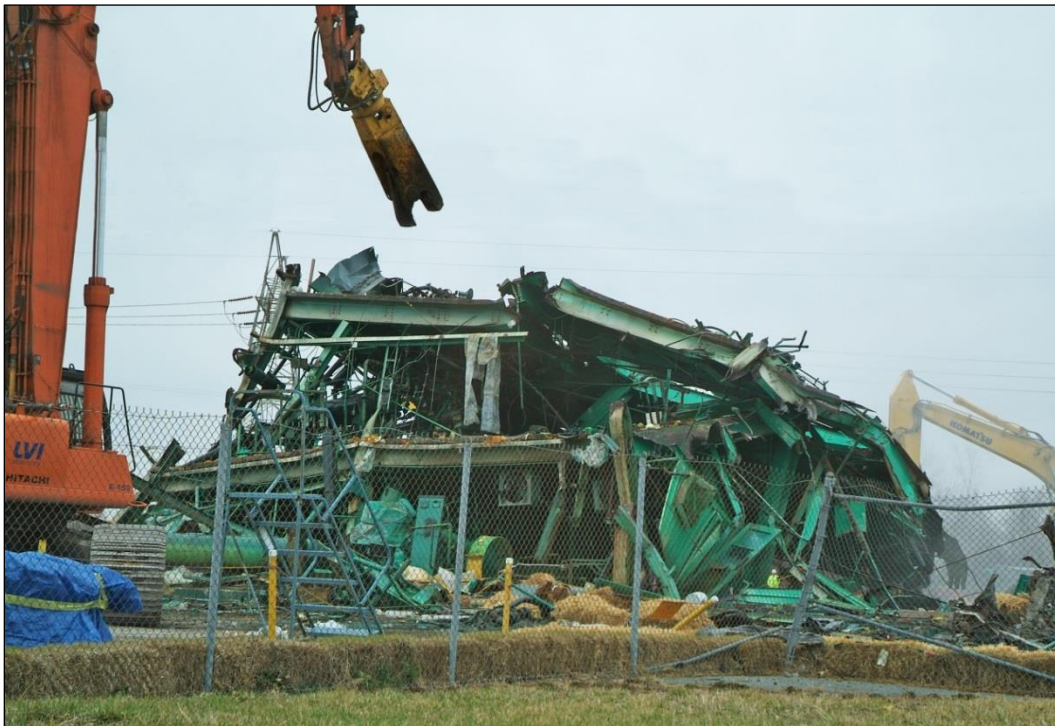
Figure A.6. The Support Beams for the Metals Plant Are Cut To Bring the Building to Slab
