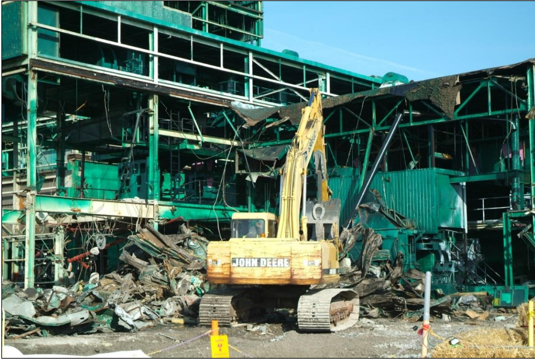
Figure A.3. Excavators with Shear Attachments Were Used to Remove Parts of the Building and Debris Generated by Demolition Activities
