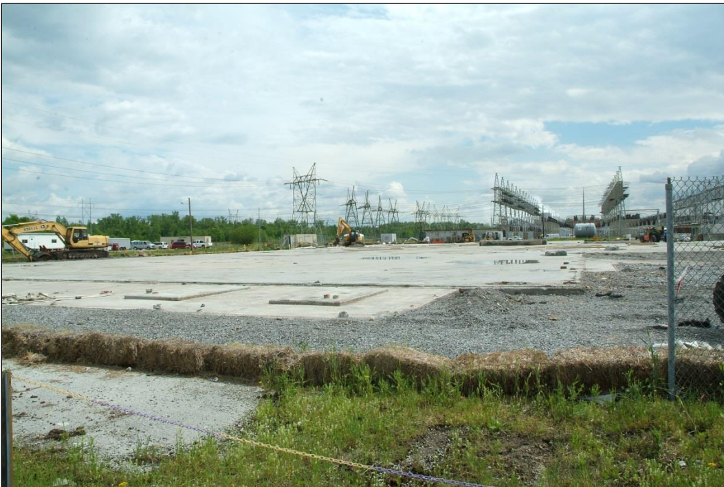
Figure A.8. C-340 Complex after Demolition
