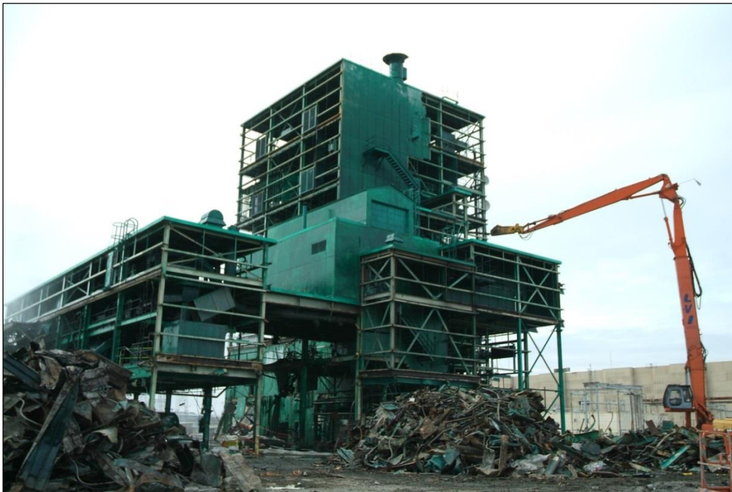
Figure A.4. An Ultra-high-reach Demolition Machine Is Used to Remove Parts of the Building That Can't Be Reached by the Smaller Excavators
