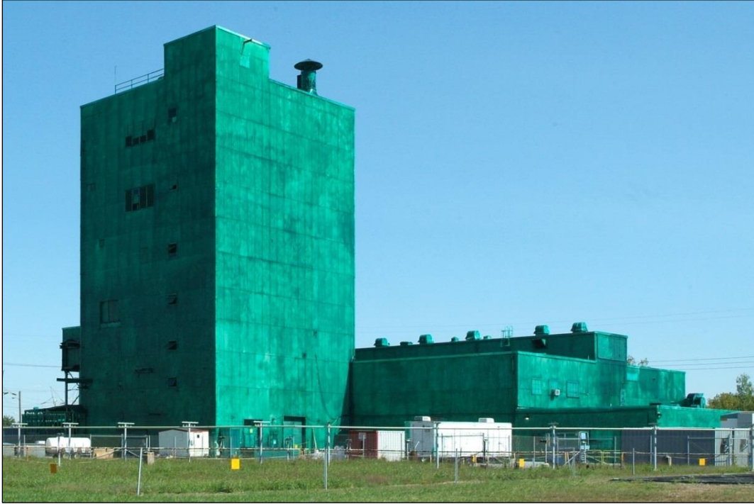
Figure A.1. C-340 Complex Prior to Demolition
