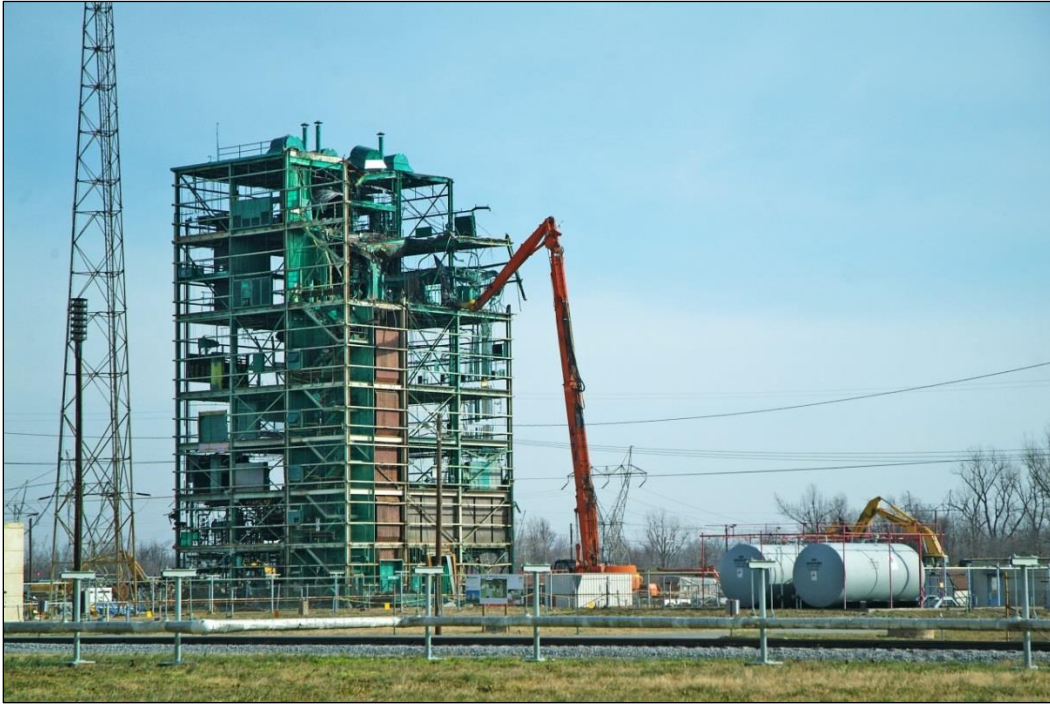
Figure A.5. An Ultra-high-reach Demolition Machine Is Used to Demolish the Metals Plant from the Top Down
