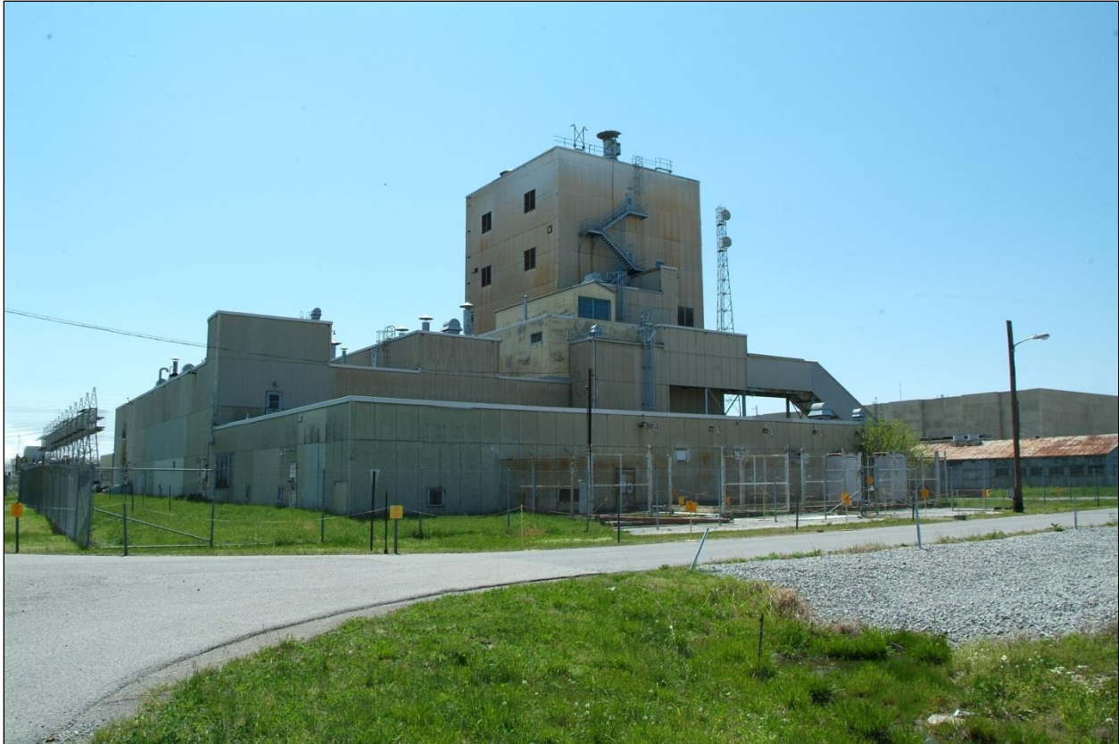
Figure 1. C-340 Complex Prior to Demolition; View is from the Northeast Corner
