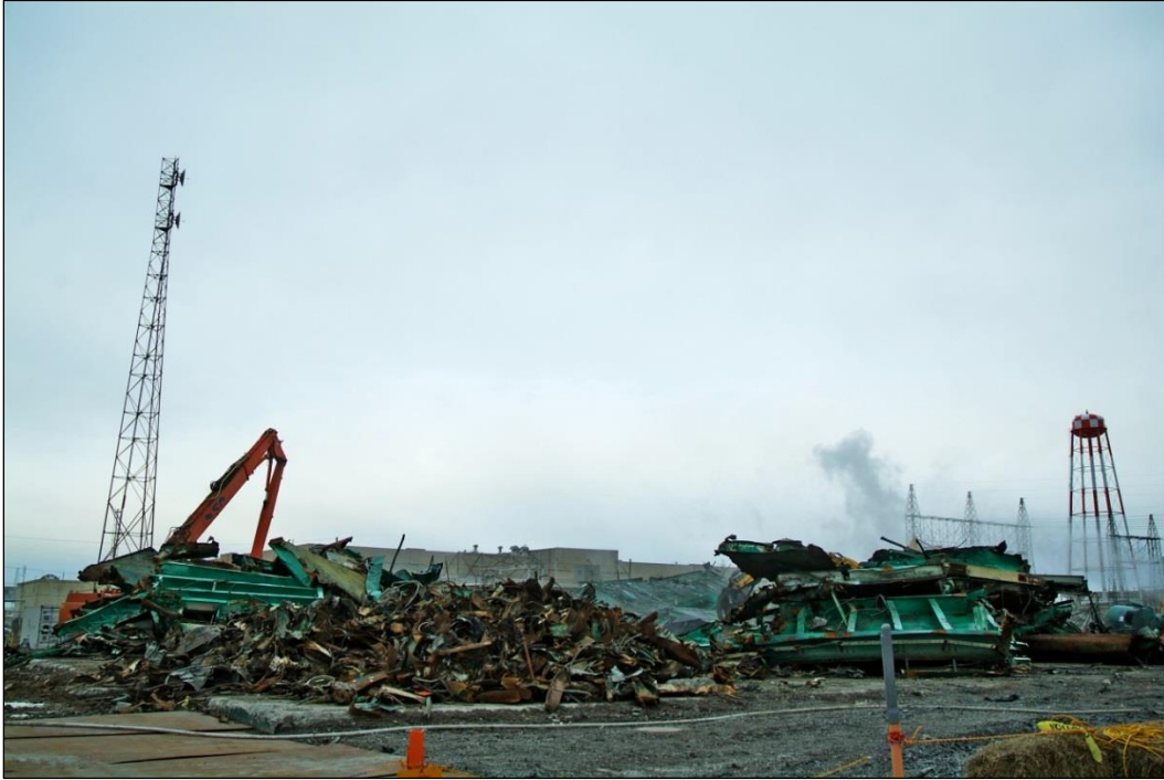
Figure A.7. Debris Is Being Sorted into Waste, Part of Which Will Be Shipped to an Approved Disposal Facility and the Rest Taken to the On-site C-746-U Landfill
